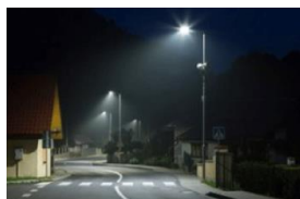
Faulty street light
