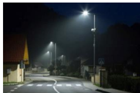
Faulty street light
