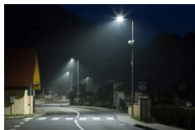
Faulty street light
